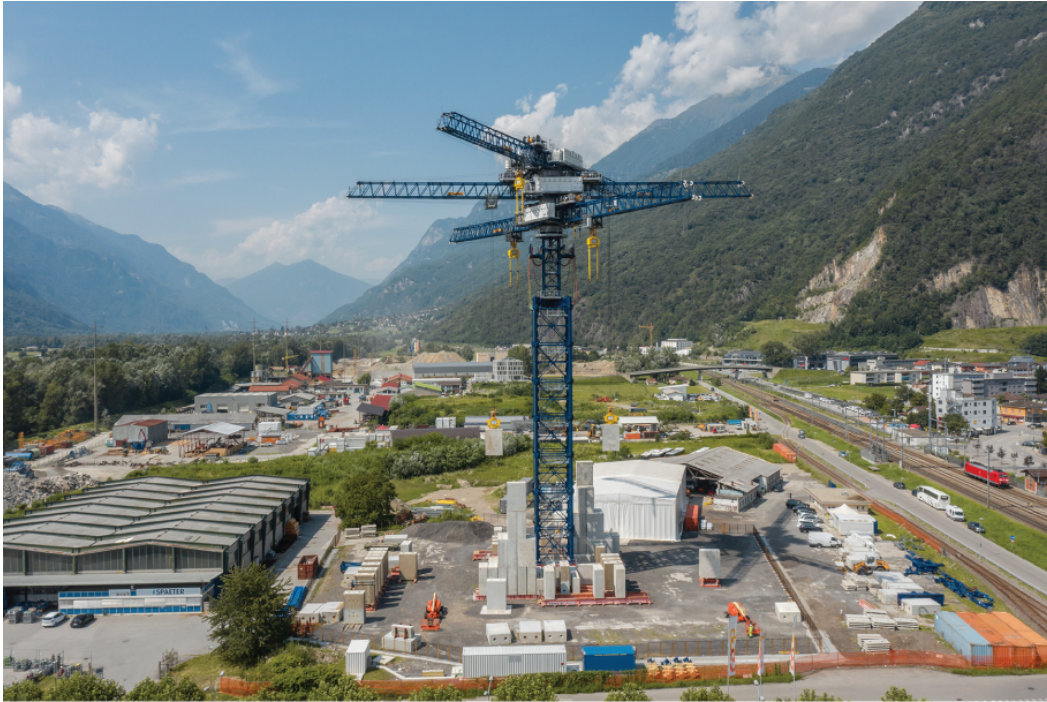
Figure 1. Energy Vault's Commercial Demonstration Unit located in Arbedo-Castione, Switzerland.
